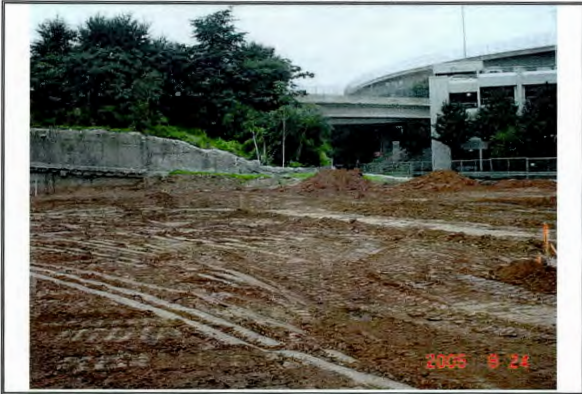
Photo # 1.: View of the graded eastern portion of the Project Site.
