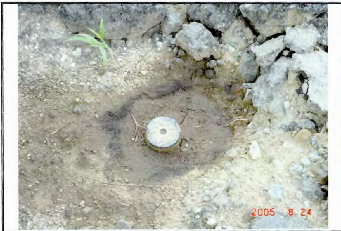
Photo # 4.: Monitoring well cap located near the southern boundary of the Project Site.
