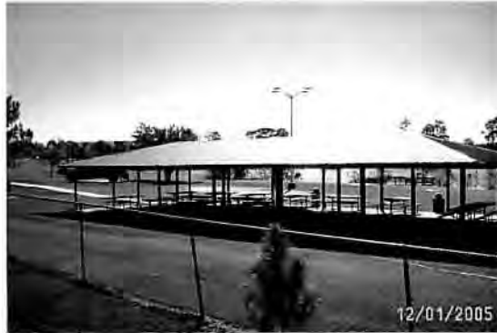
Photograph 10 Pavilion located at the southwest end of the site.
