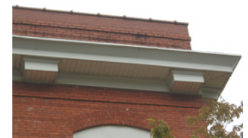
Figure 30. On Tift Hall, the original wood cornice and mutules (box-shaped projections) have been covered with corrugated vinyl fascia which detract from the historic character of the building. On Herring and Lewis Halls, the mutules have been completely removed.
