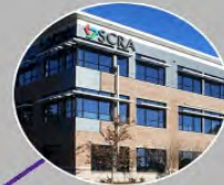
SCRA Applied Technologies Center (Summerville Building)
