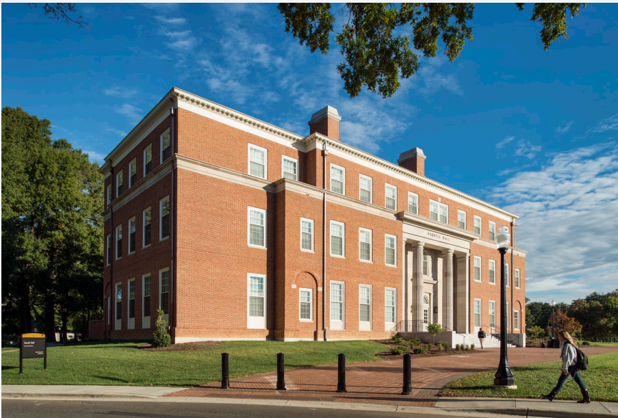
Farrell Hall's traditional brick exterior maintains continuity with the other buildings on the Wake Forest campus.
