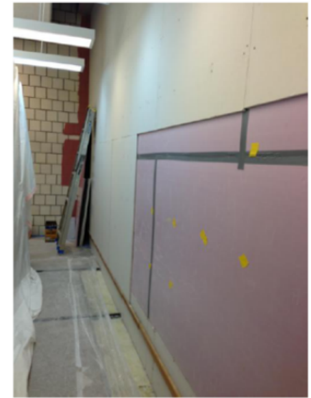
Insulation and drywall applied to Room #1
