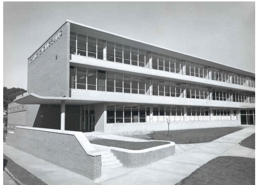
Textile Engineering Building-GIT (1946)
