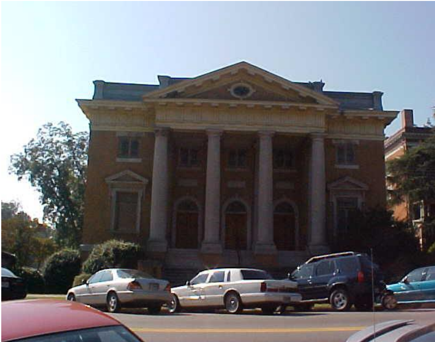
Former First Methodist Church Building—GCSU Before Renovation (2003)
