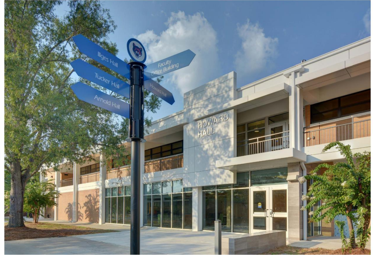
Howard Hall-Columbus State University Rear Façade--After Renovation (2016)
