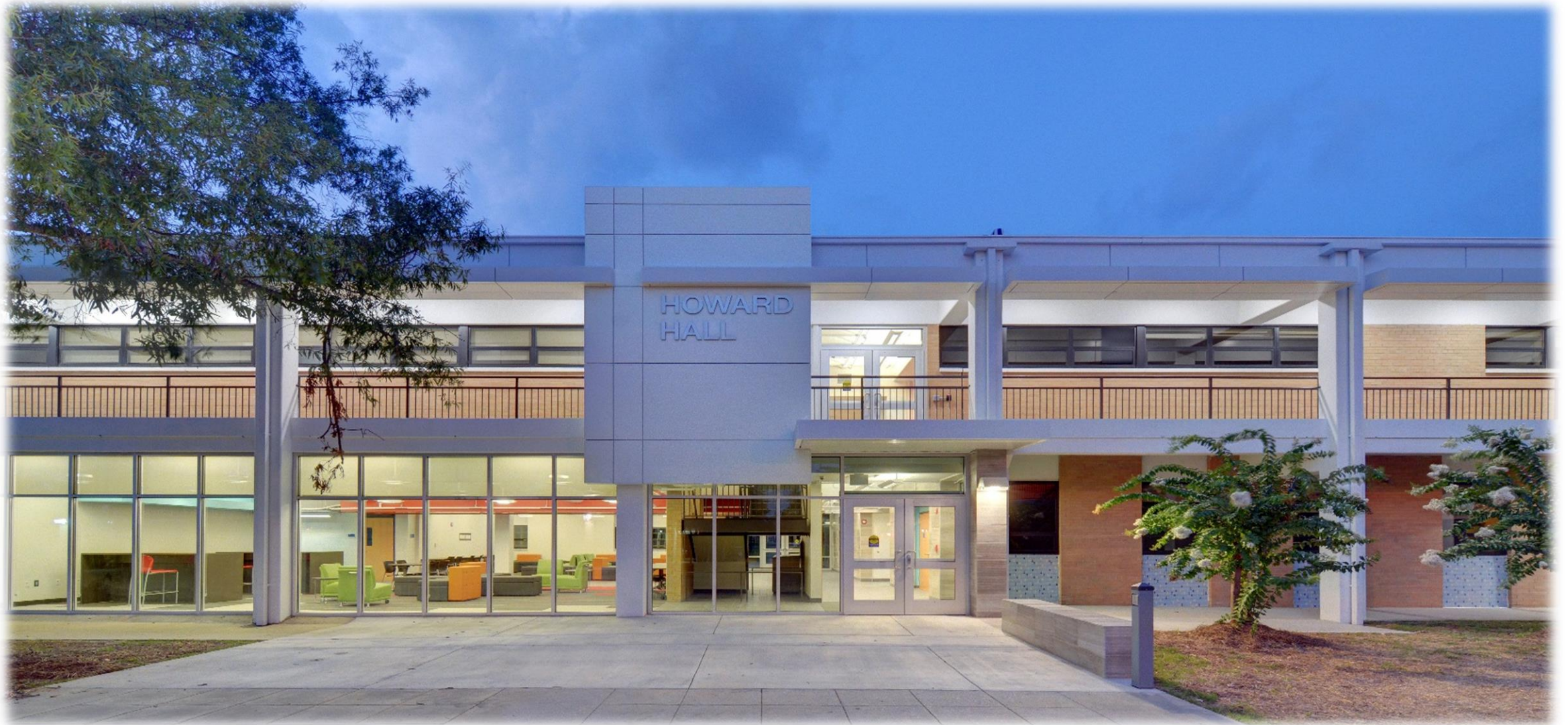
Howard Hall-Columbus State University Rear Façade--After Renovation (2016)
