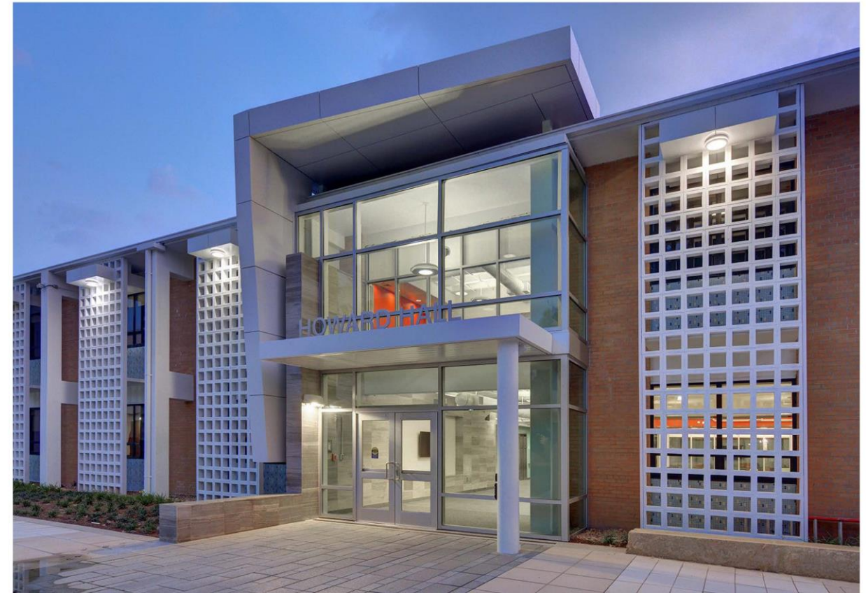
Howard Hall-Columbus State University Front Façade--After Renovation (2016)
