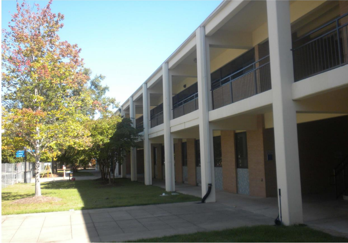
Howard Hall-Columbus State University Rear Façade--Before Renovation (2014)
