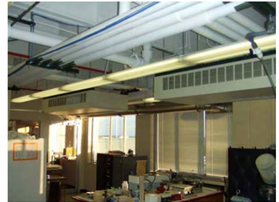
Lab with Exposed Fan Coil Units
