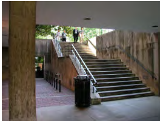
Stairs provide the only exterior grade transition from the lower level in front of the Hinman Building to the main entrance level fronting on Cherry Street.
