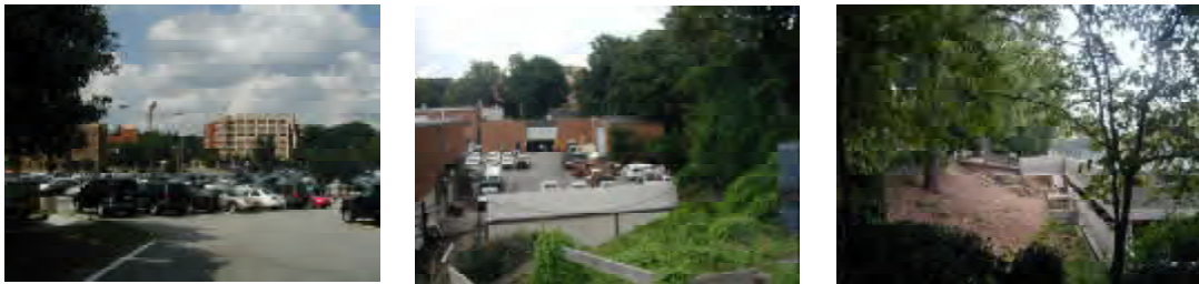
Figure 18 Required Demolition for the Eco-Commons; L-R: Parking west of Hemphill, Physical Plant, and the Peters Parking Deck.
