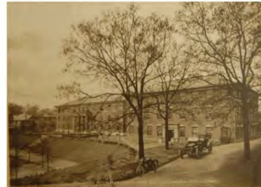
Savant and Swann Buildings: note service lanes, Savant and Swann plaza, hedge along service lane, stairs to Swann, and mature trees along service lane (c.1910)
