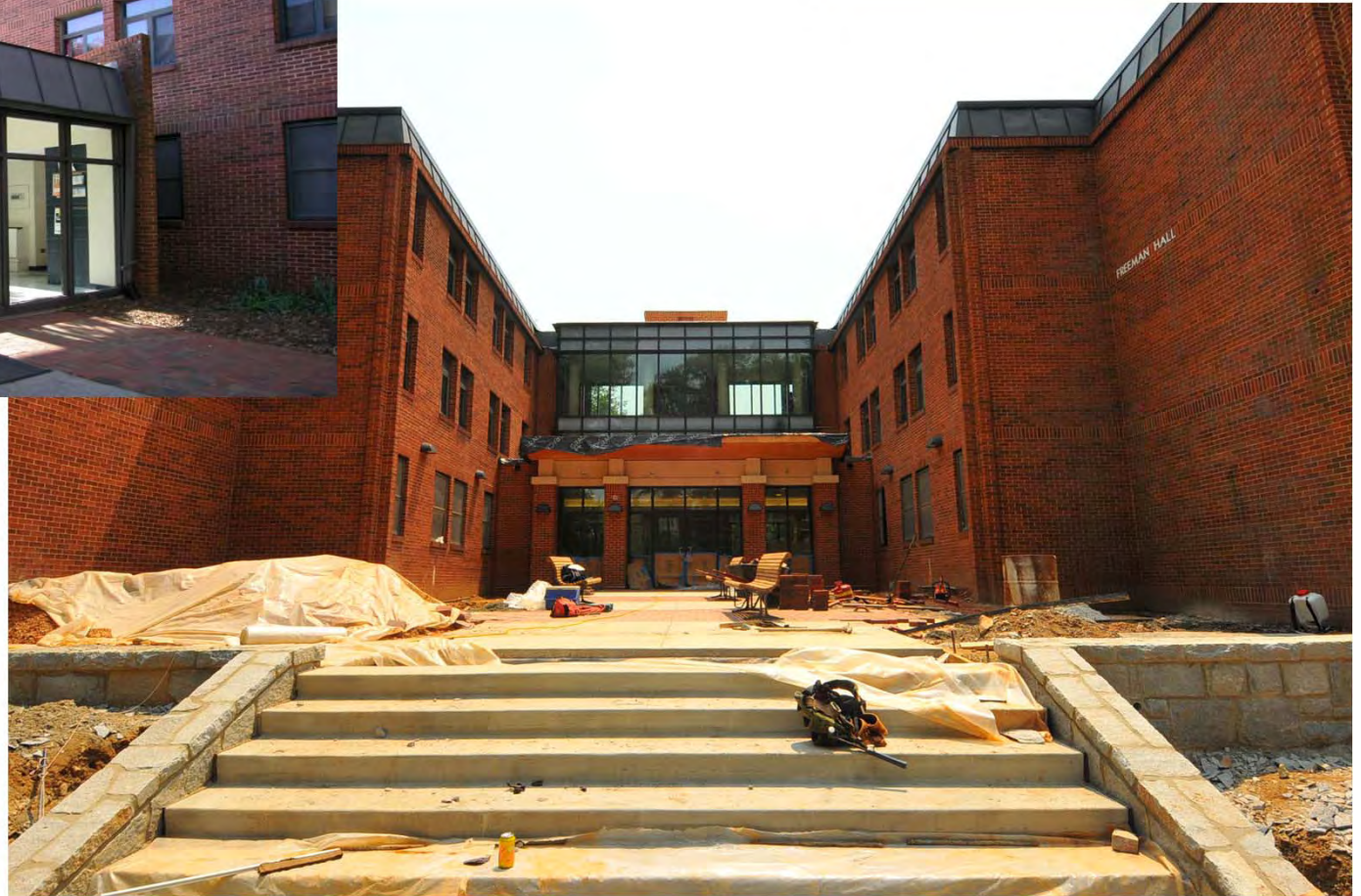
Exterior Front Entrance - after
