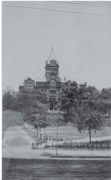
Administration Building and Service Lane: note service lane street trees, service lane alignment, adjacent slopes to service lane, and recently planted hedge (c.1910)
