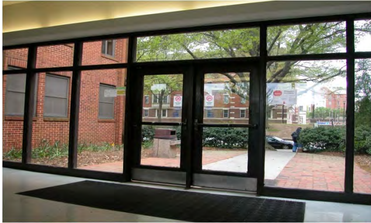
Interior Entry Looking Out - before
