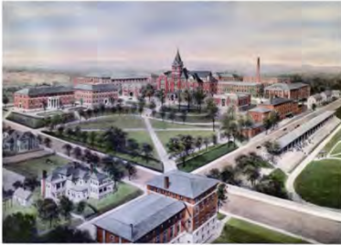
Bird's Eye View of Tech Tower Lawn : note hedges, street trees, service lanes, sidewalks, and Savant and Swann plaza (c.1920)
