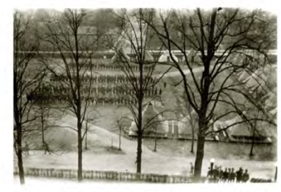
Tech Tower Lawn: note cruciform sidewalks, young hedges, large white oak, young street trees, and offset stairs and sidewalk (c.1918)
