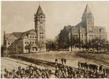
Shop Building and Administration Building: note trees in front of Administration Building (c.1888)
