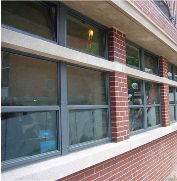
Restored Windows w/ Insulated Glass
