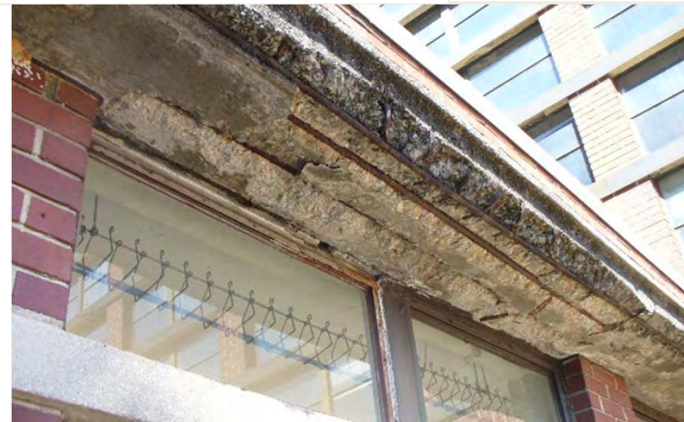
Cast In Place Architectural Concrete
