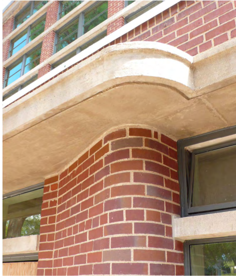
Restored Architectural Cast in Place Concrete
