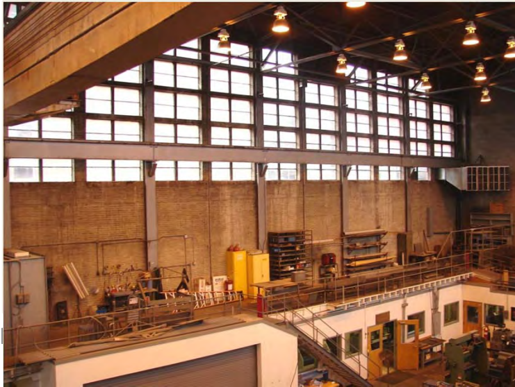
Inadequate Resistance to Sheer
