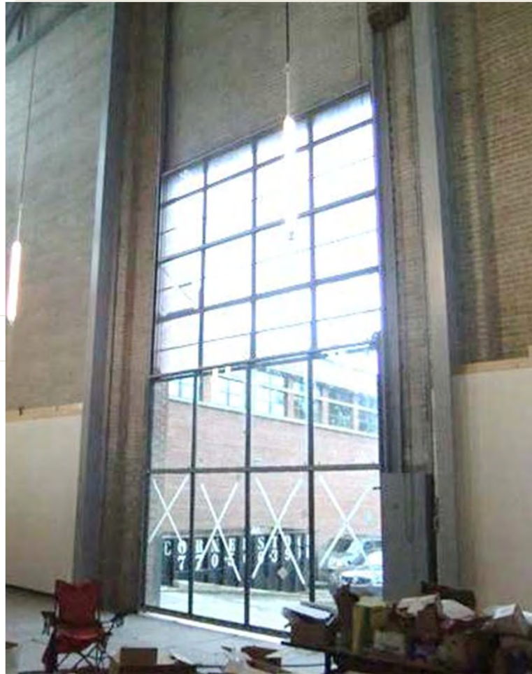
Supplemental Steel Framing
