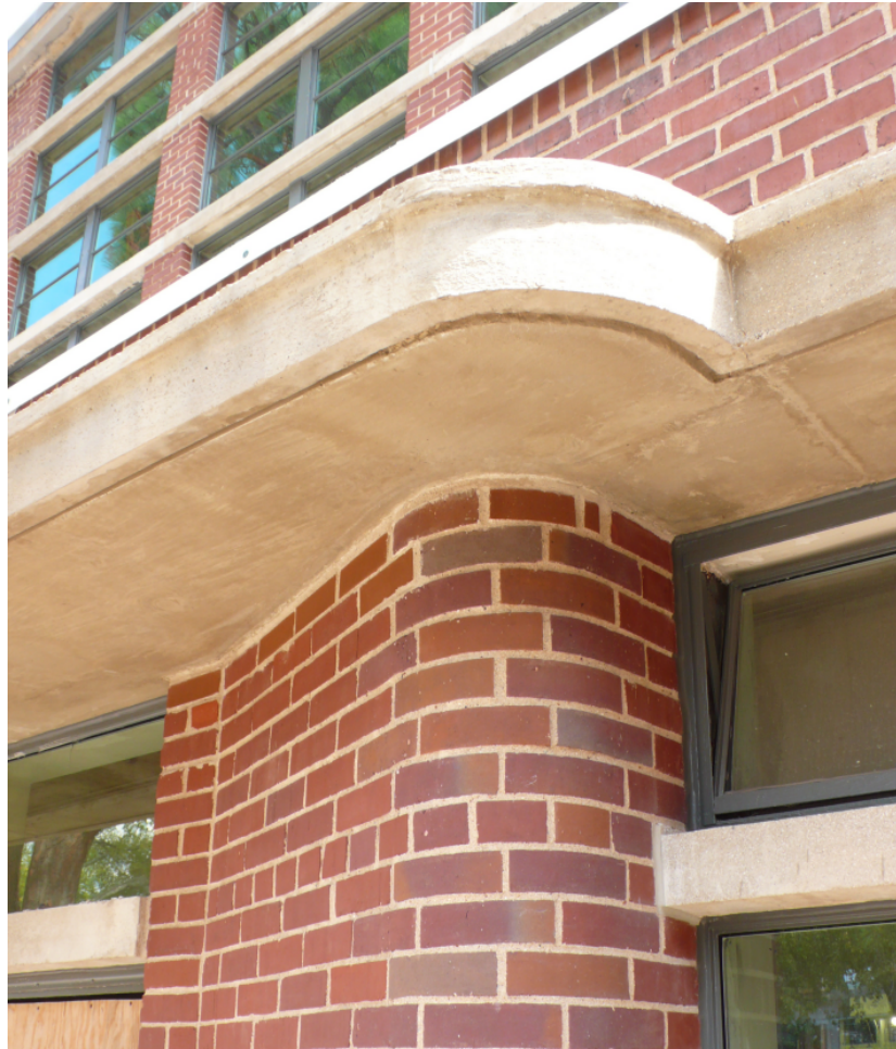
Restored Architectural Cast in Place Concrete
