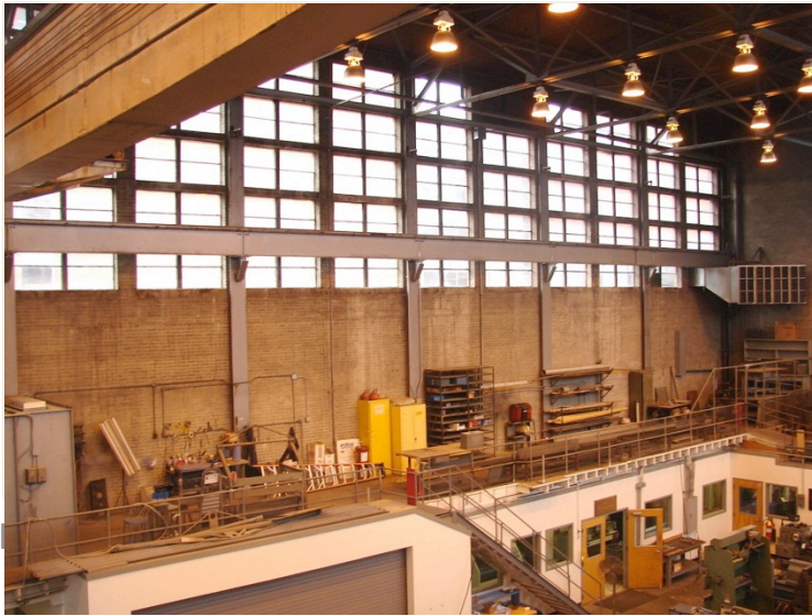
Inadequate Resistance to Sheer
