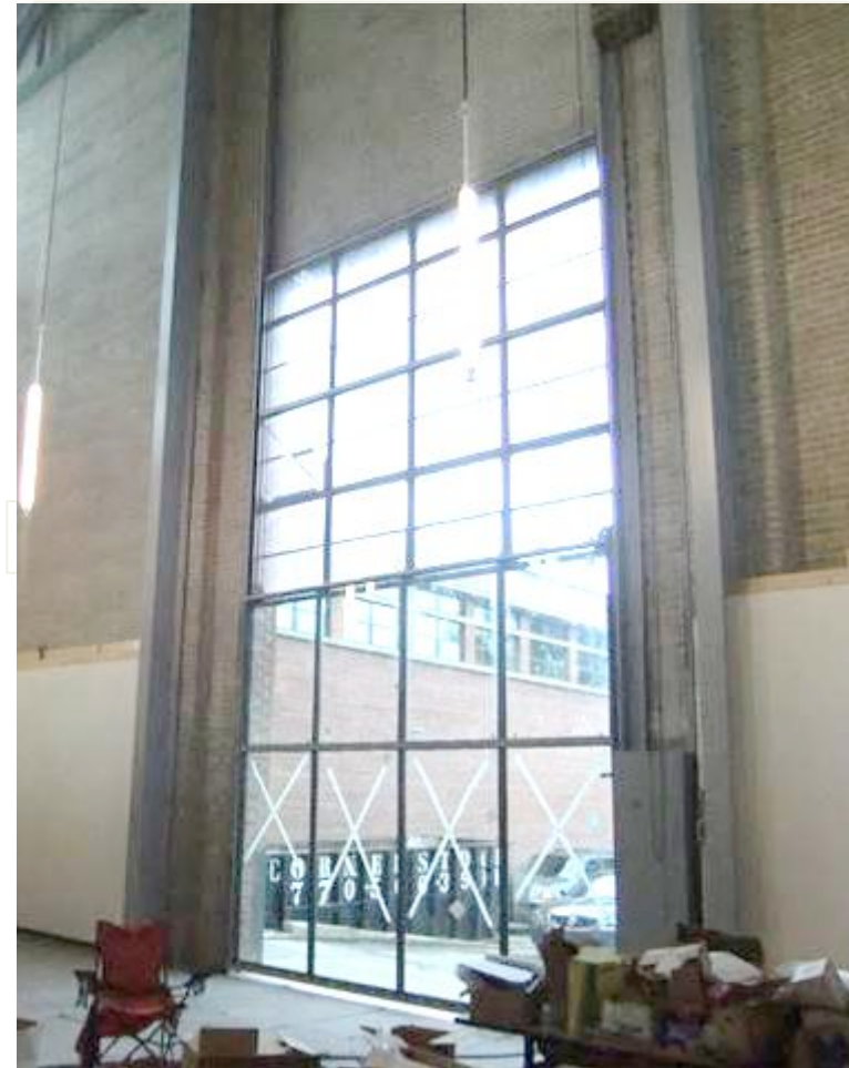
Supplemental Steel Framing
