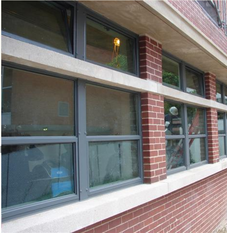
Restored Windows w/ Insulated Glass
