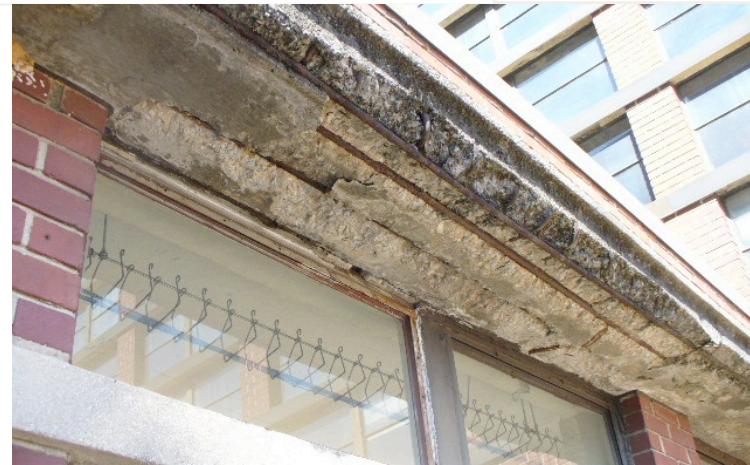
Cast In Place Architectural Concrete
