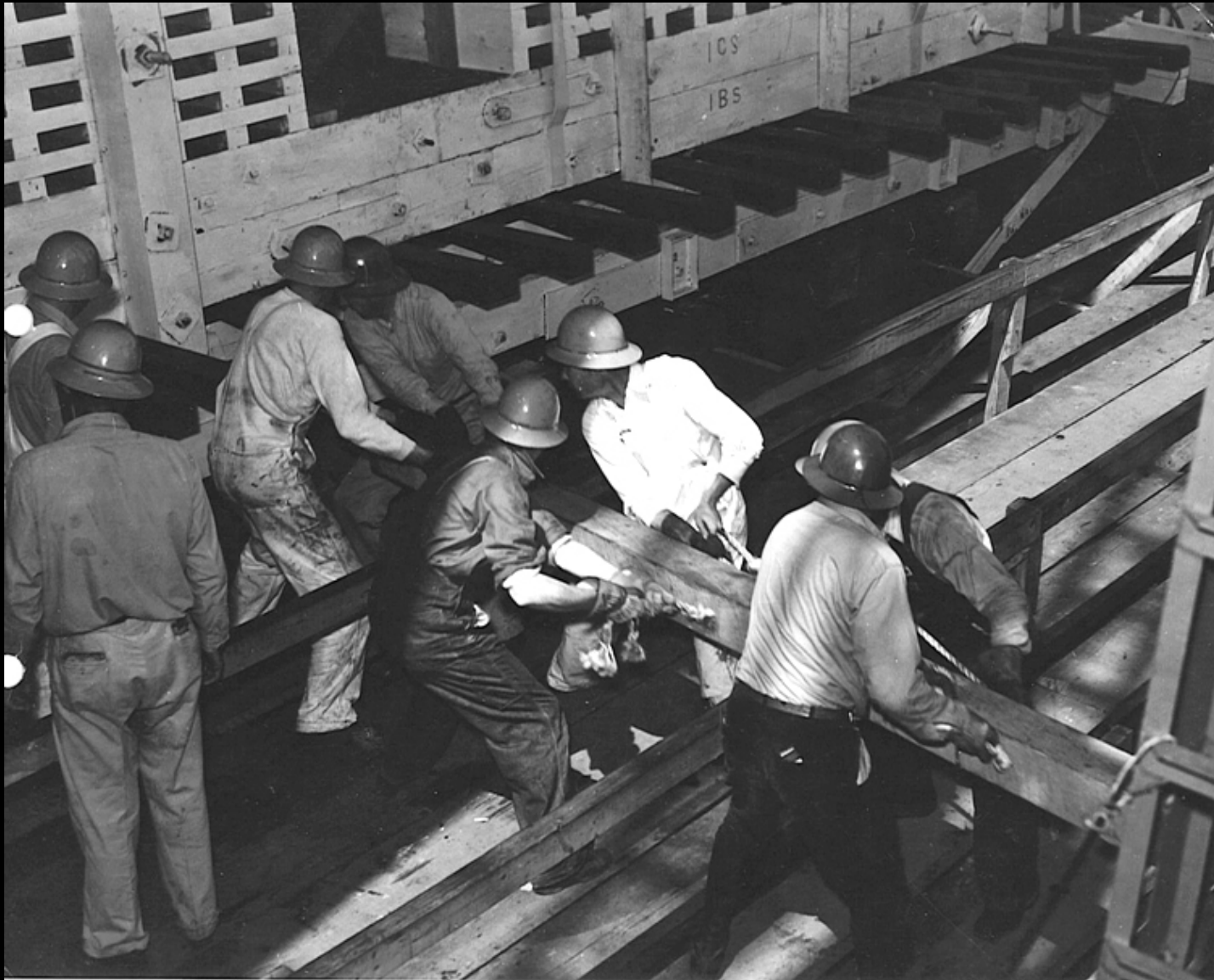
Pulling wedge beneath hull (jaj109)
