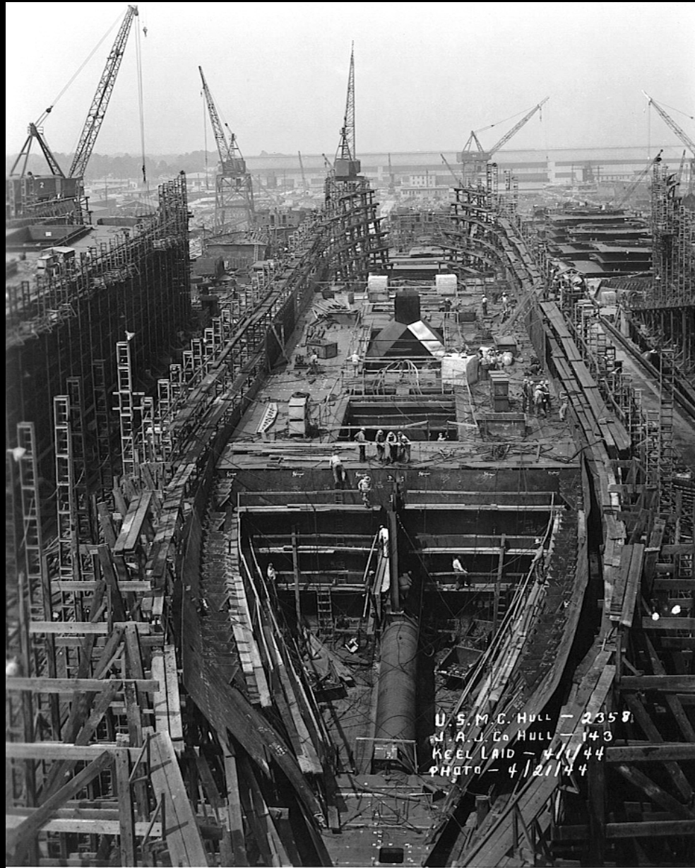
Shaft tunnel in hull [Samlorian] (jaj011)
