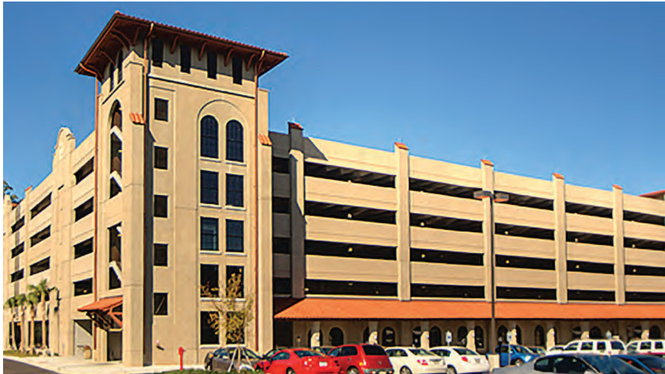
Existing Parking Structure
