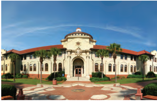
West Hall constructed in 1917
