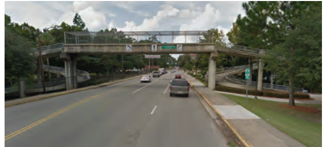
Pedestrian overpass on Oak Street
