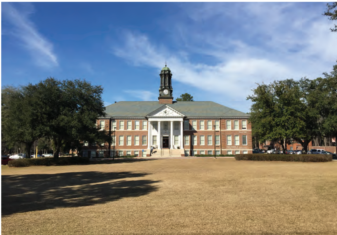
Pound Hall, North Campus
