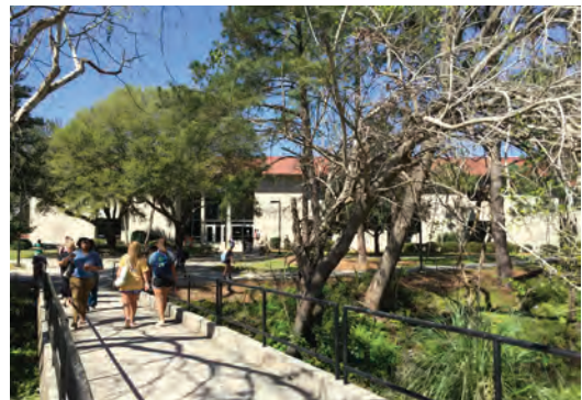
Existing pedestrian bridge on One Mile Branch
