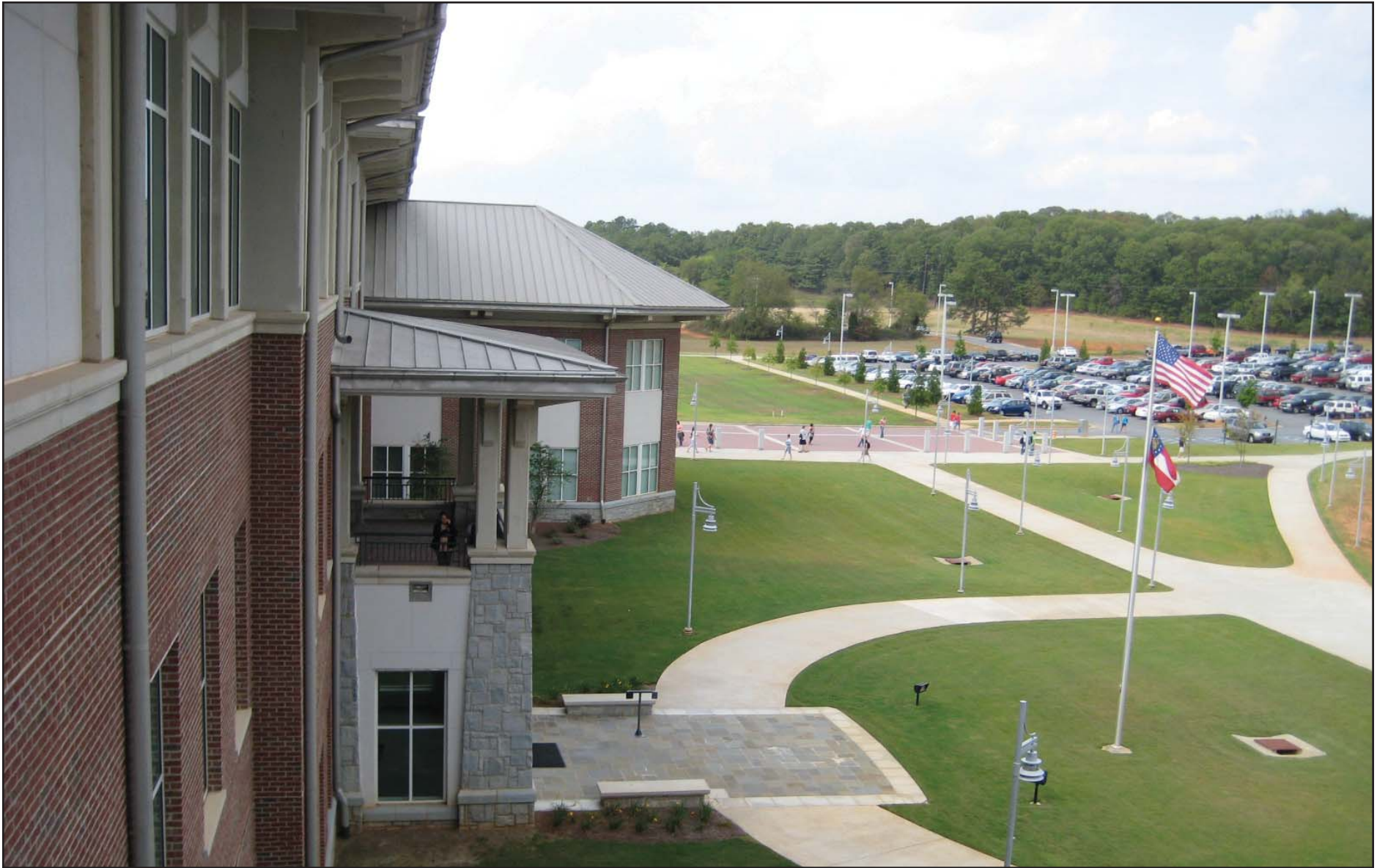
VIEW OF THE BARTOW CAMPUS ACADEMIC BUILDING AND ASSOCIATED PARKING
