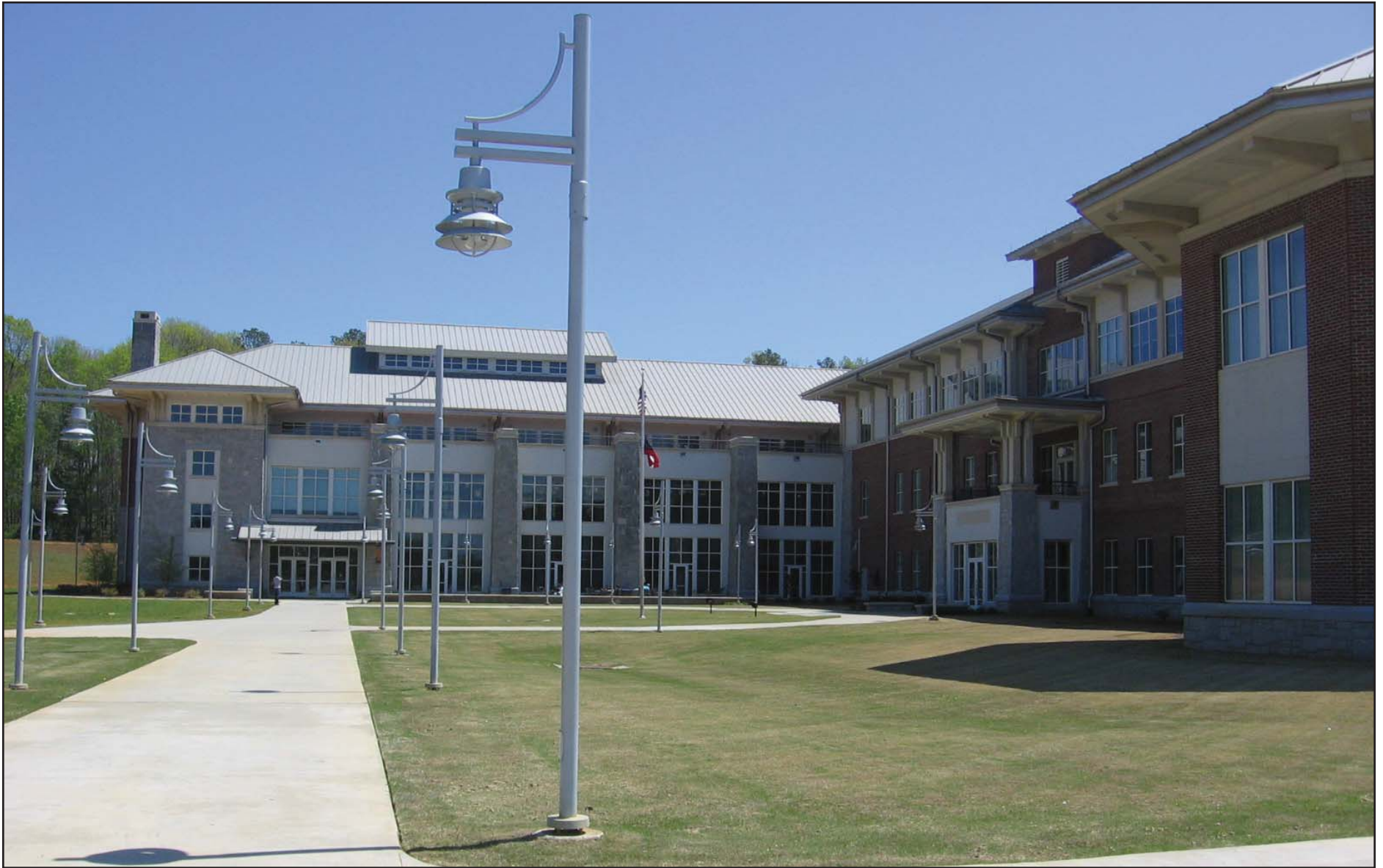
VIEW OF THE BARTOW CAMPUS ACADEMIC BUILDING
