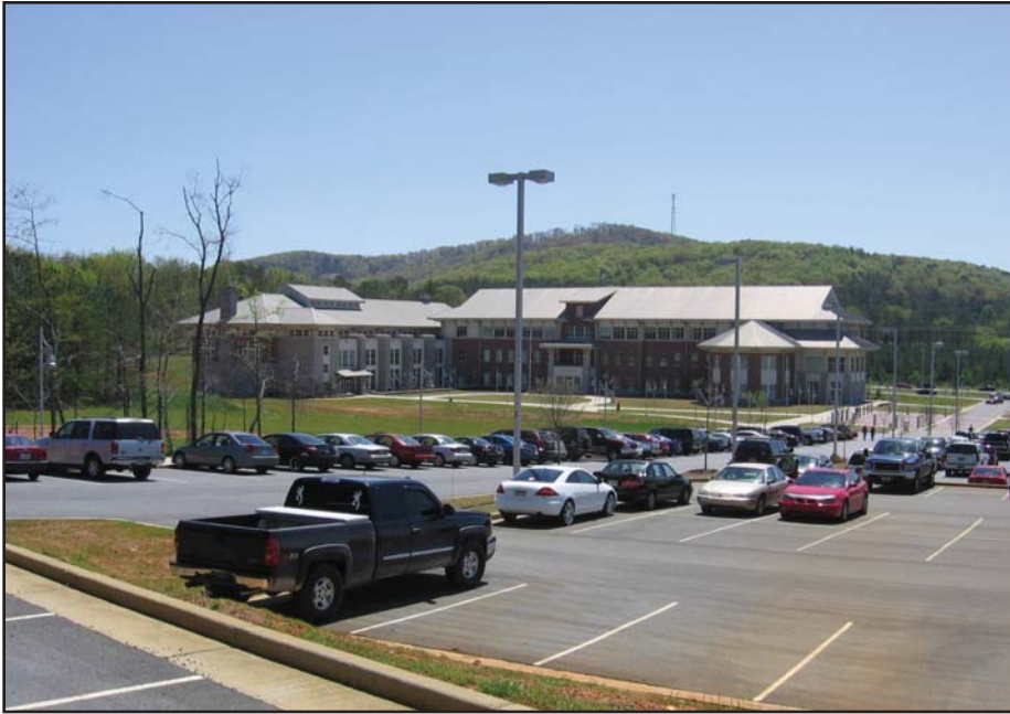
VIEW OF THE ACADEMIC CORE FROM THE NORTH
