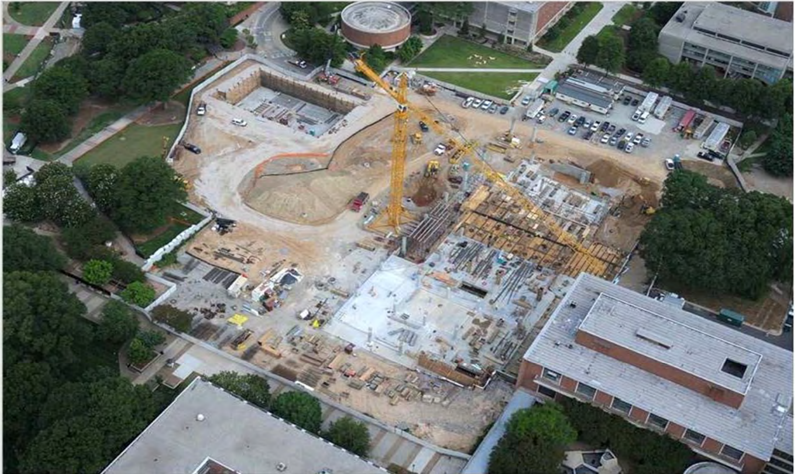
Central Campus Cistern – 1.4 million gallons
