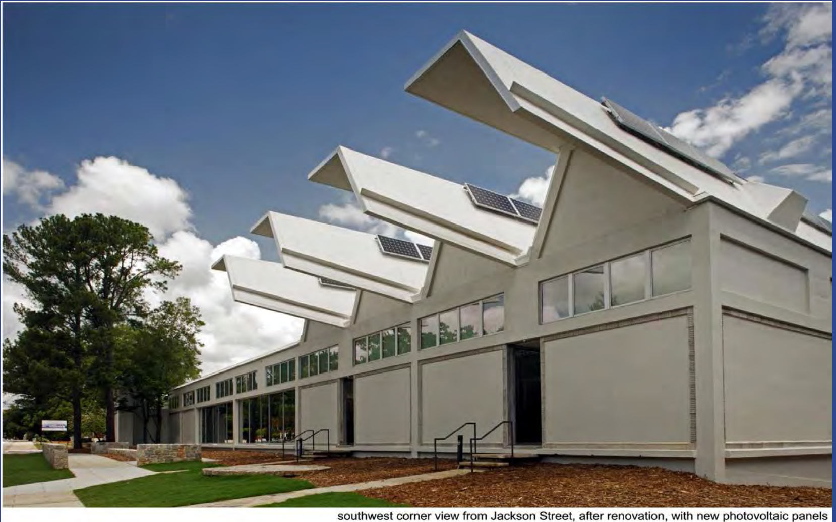
southwest corner view from Jackson Street, after renovation, with new photovoltaic panels
