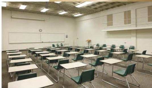
former high-bay classroom (before renovation)
