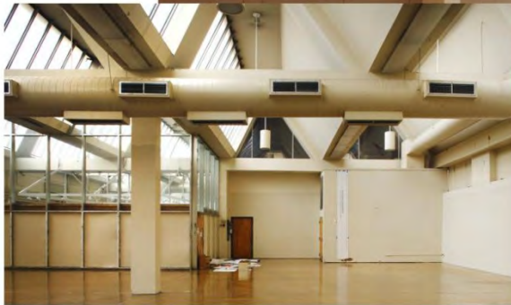
former high-bay studio space (before renovation)
