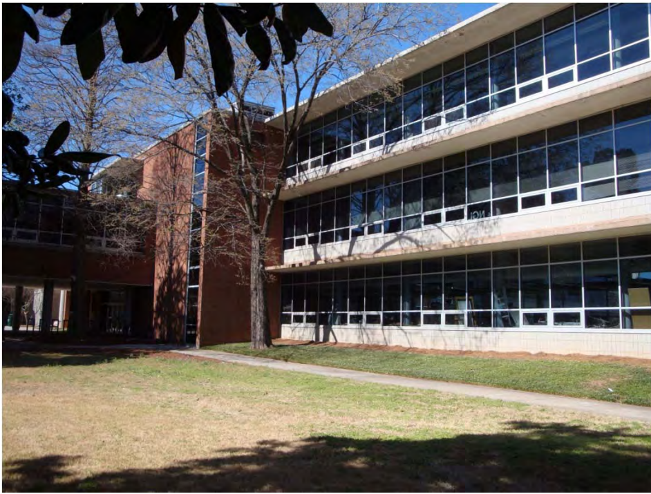
Architecture Bldg, courtyard, south elevation
