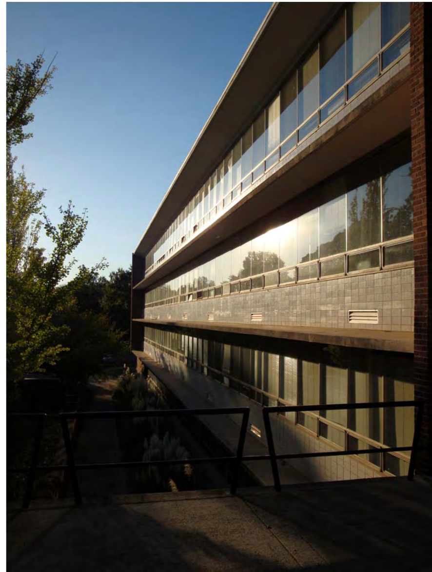
Skiles Classroom Bldg, south elevation
