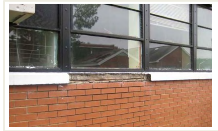
Window and masonry rehabilitation
