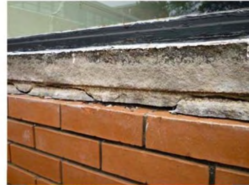
Miller Building – crack on the outside wall from outside
