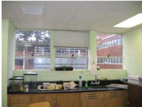
Miller Building - labs steel windows from inside view
